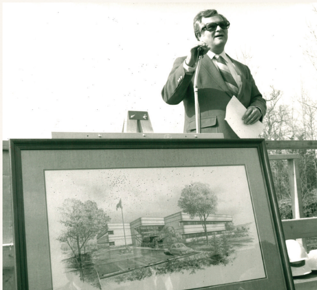
Former CATIC president L. Stewart Bohan breaks ground for CATIC’s building in 1982.
